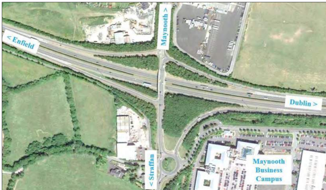
Figure 4.9: Junction 7 Maynooth – Aerial (© Google Imagery ©2020 DigitalGlobe)
