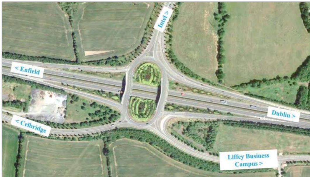
Figure 4.5: Junction 6 Celbridge – Aerial (© Google Imagery ©2020 DigitalGlobe)
