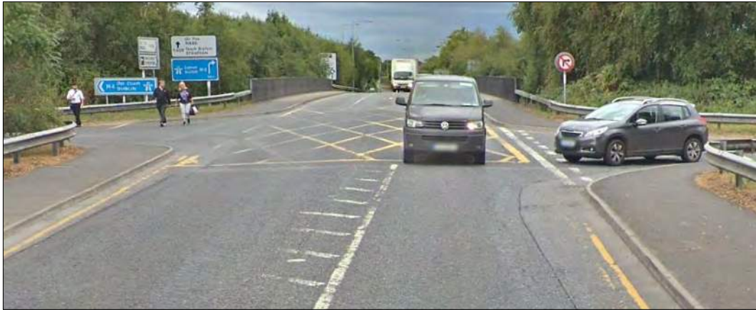
Figure 4.7: Vulnerable Road Users at Junction 7 (©2020 Google)
